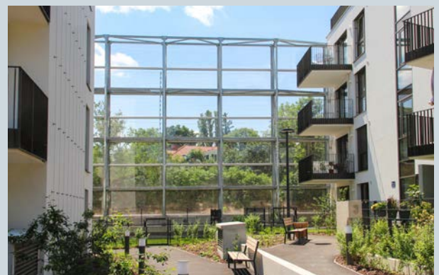
Noise screens ensure tranquillity: a courtyard in Vienna's 13th district is protected from traffic noise.
