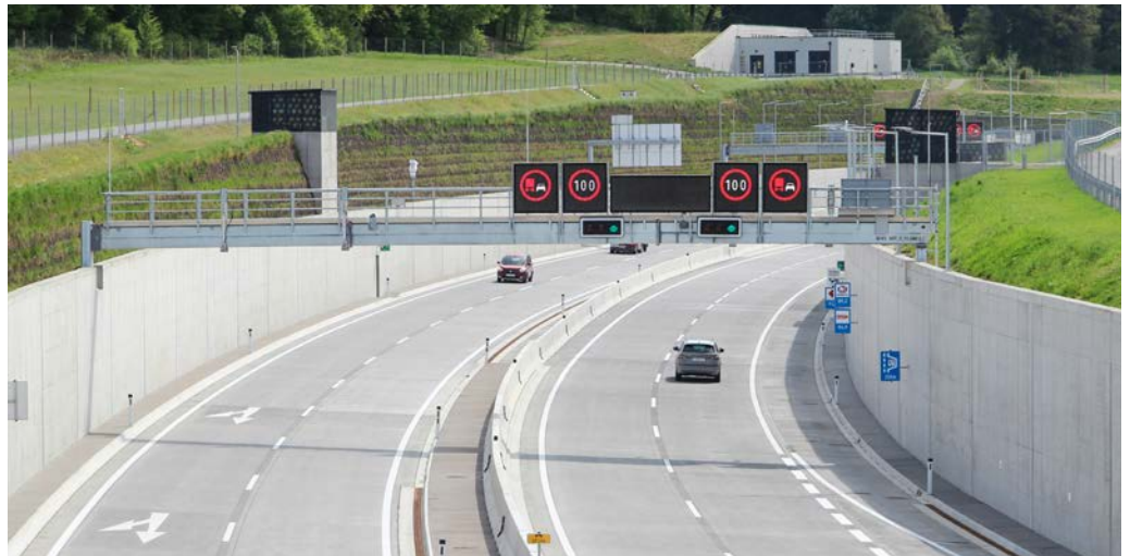
The subsurface structure required special designs for the gantries.
